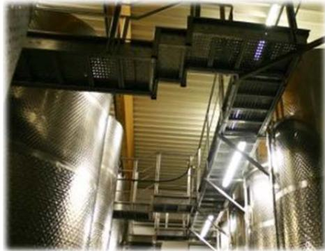
Walk-on gratings can be combined into platforms, walkways, staircases, overhead passages and other walk-on surfaces. These walk-on structures can be used in any facilities (industrial plants, wine cellars, etc.), where a safe and convenient access to difficult elevated locations is required.
